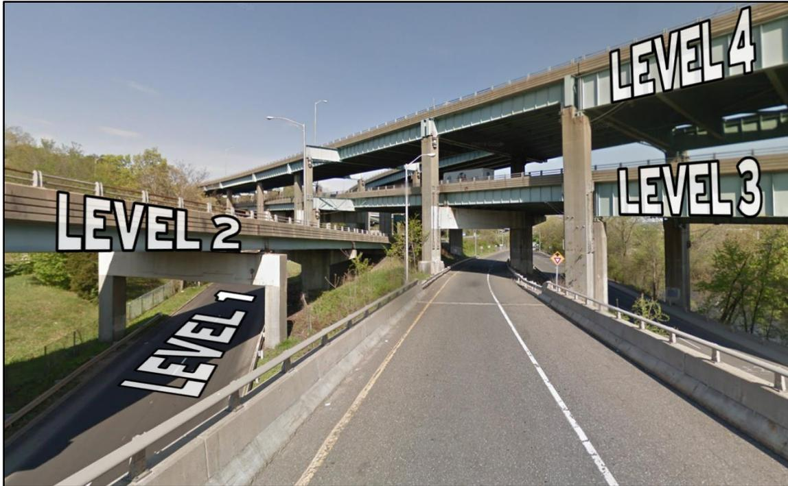
Figure 2-3. Stacked Mixmaster Interchange Structure with Four Levels
